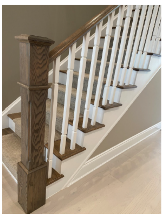
Split Finish Staircase
